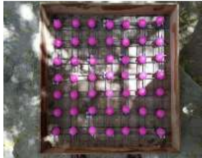
Fig 7: Reinforcement and HDPE ball arrangement
