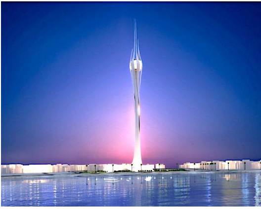
Figure 9. Overall view of the tower
