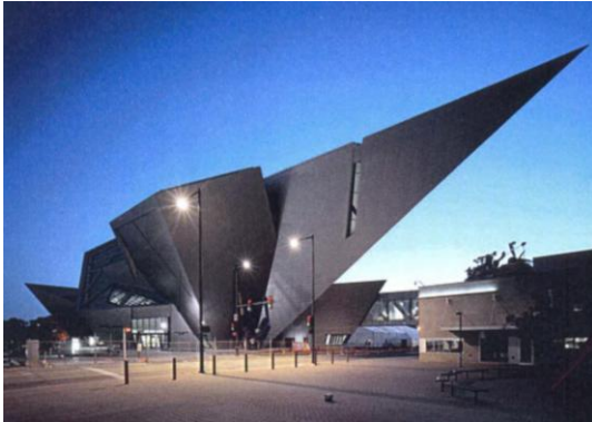
Figure 2. The Hamilton Building (Denver Art Museum Extension)
