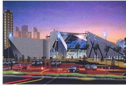
Figure 8. Front view of the exhibition center
