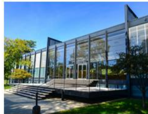
Figure 2. S.R. Crown Hall, IIT, Illinois [7]
