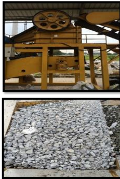
Figure 1 & 2. Process of crushing the waste cube into recycled concrete aggregate
