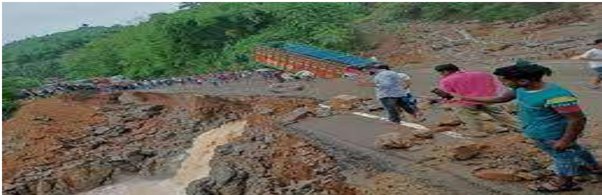
Fig. 4 - Flood damage on NH6 in Meghalaya, India, June 2022
