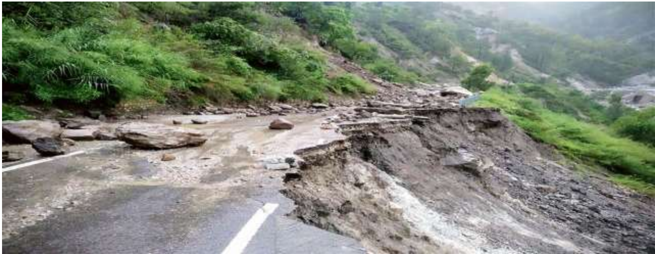
Fig. 5 - The Shimla-Kinnaur road damaged due to a landslide
