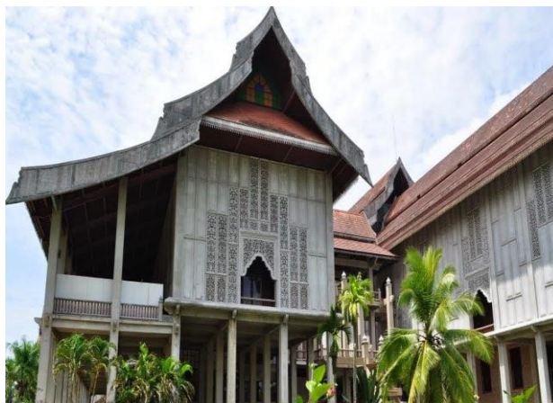
Figure 5: Example of concrete wall with traditional aesthetic elements applied at Terengganu State Museum
