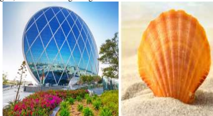
Figure 5. (a)Aldar Headquarters,UAE (b)Shell
