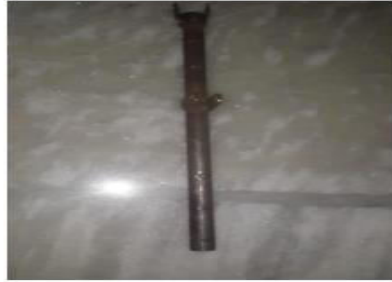
FIG 8 FABRICATION OF VERTICAL MEMBER
