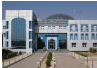
Arches for aesthetic purposes only, Ministry of Awqaf/Endowment and Religious Affairs, Erbil, Kurdistan Region of Iraq
