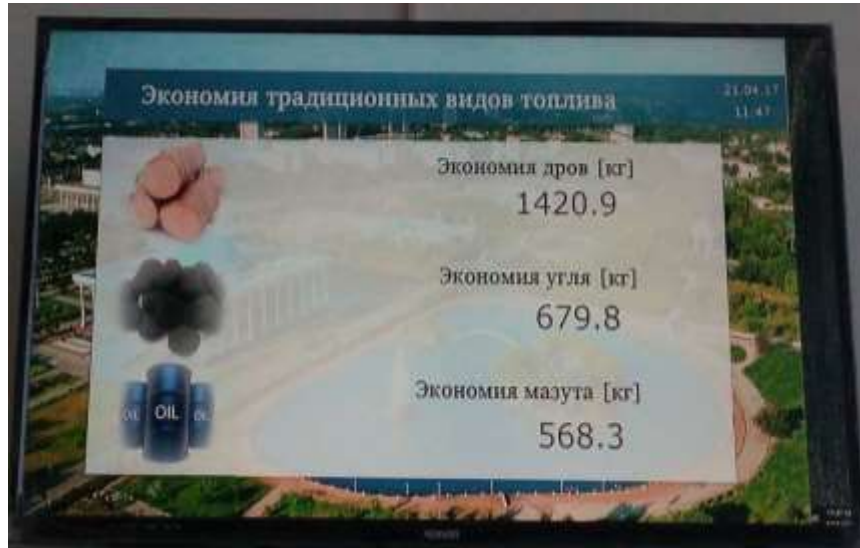
FIGURE11. Monitor for presenting daily and monthly parameters of the PVS (as of 21.04.2019)
