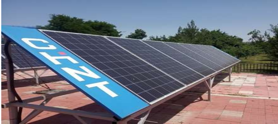
FIGURE 1. General view of a solar photovoltaic station with a capacity of 10 kW
