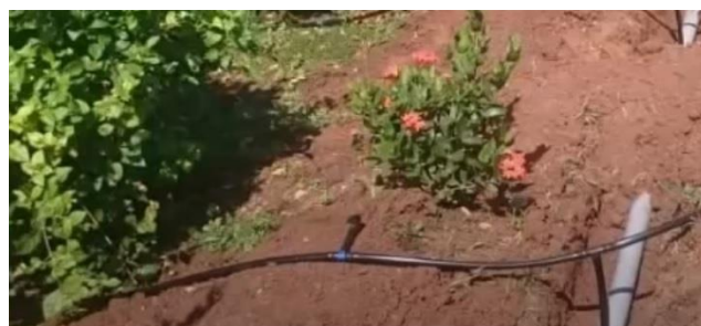
Figure 6. Drip Irrigation System with HL Value.
