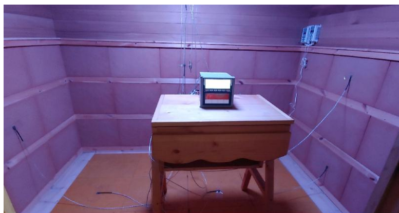
Fig. 4 A diagram of installation of temperature sensors for measurement of air temperature and wall surface temperatures inside a small two-person pension
