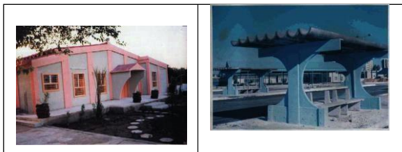
Figure 9: Buildings constructed with ferrocement
