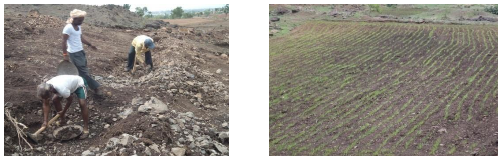
Photo 2: Inter-cropping Pattern and Constructed Contour Trenching
