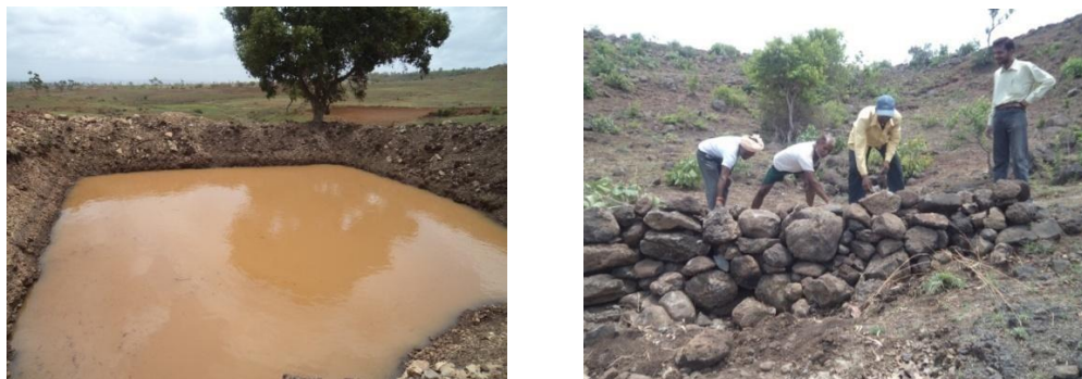
Picture 1: Built Farm Pond and Gully Plugs
