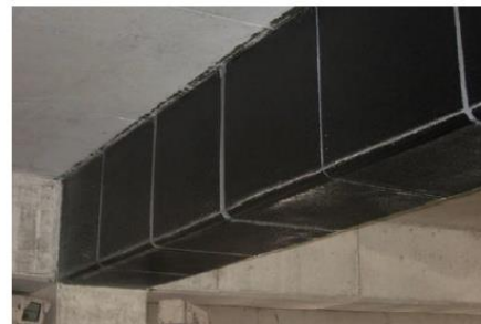
Figure No. 3 Carbon FRP fiber installation
