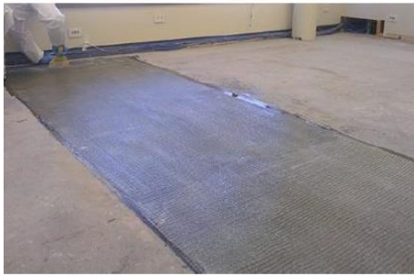
Figure No. 4FRP Composite Strengthening services Concrete solutions
