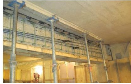
Figure No. 1 External Post Tensioning
