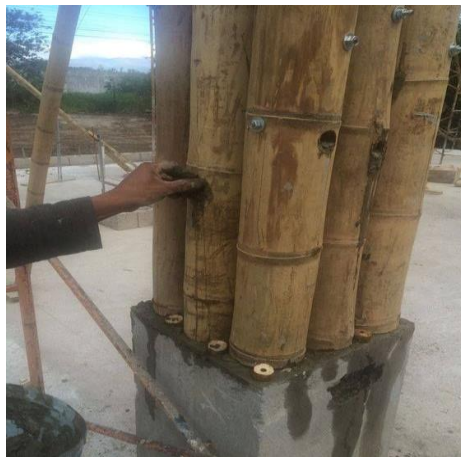
Fig. 1 Bamboo reinforcement in columns
