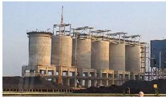
Figure 1: RCC Group Silos
